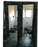
PIANO PRIMO IN DISUSO
