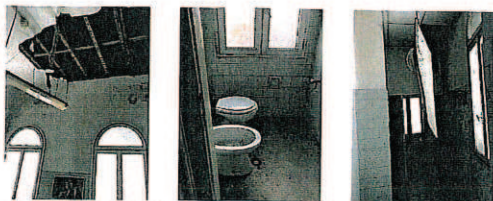
PIANO PRIMO IN DISUSO
