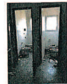
PIANO PRIMO IN DISUSO
